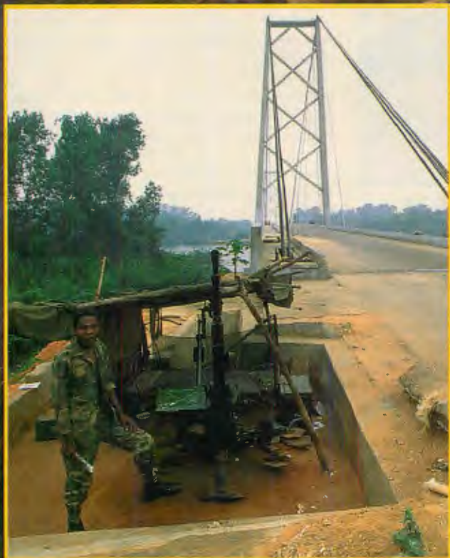
Because of the security threat, the Angolan government has found it necessary to guard every bridge in the country, such as this one over the Cuanza, south of Luanda.
